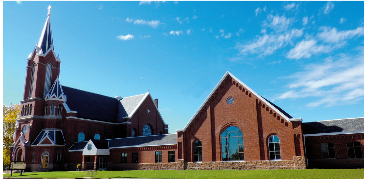
The new parish center at the Church of St. Anthony in Watkins is located just to the north of the church on Central Ave. It boasts a large main dining hall, offices, a kitchen, an elevator for handicap accessibility, and five classrooms for faith formation. (Photo courtesy of the Church of St. Anthony)
